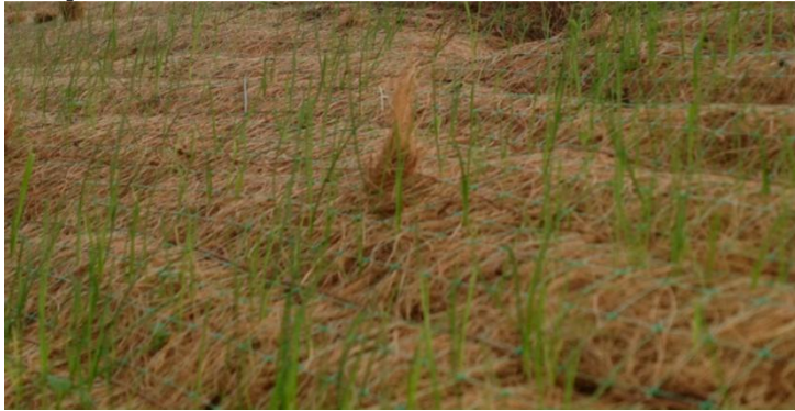
Covamat Fresh by Greenfix, immediately after installation
